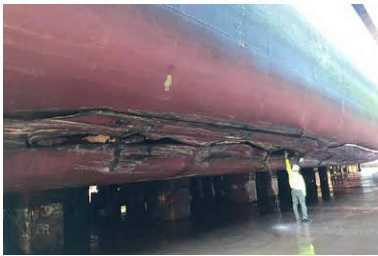
Damage to Seatruck Performance port side.
