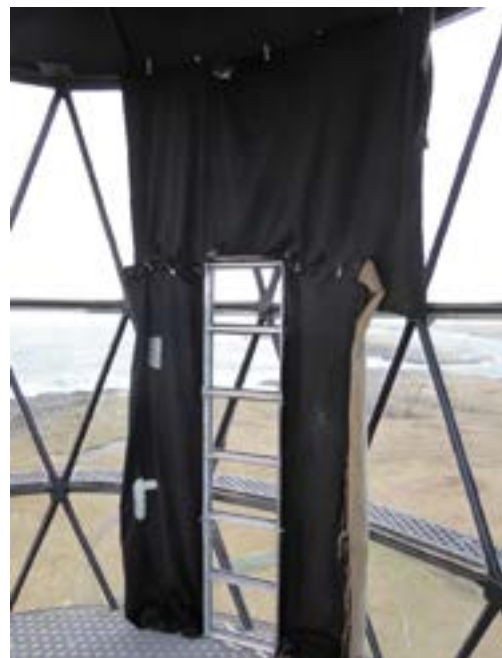
Figure 3 – Prisms frames temporarily installed at a lighthouse
