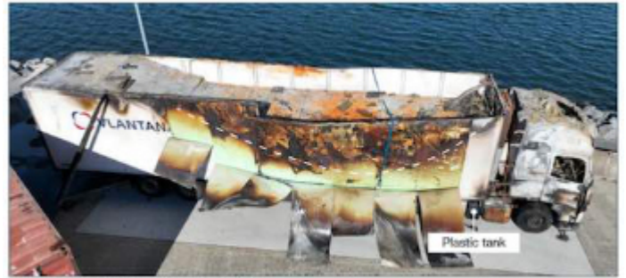
Figure 18: Fire pattern on the truck's right side. Source: DMAIB
