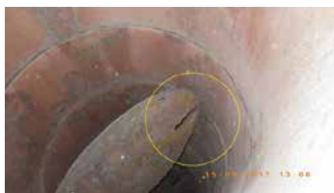
Defective fire damper.
