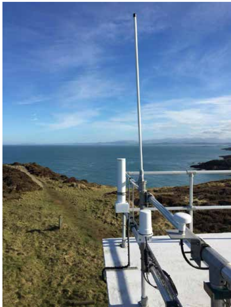
Antenna Installed at Point Lynas former Fog Signal building showing VHF, GPS and 4G antenna.
