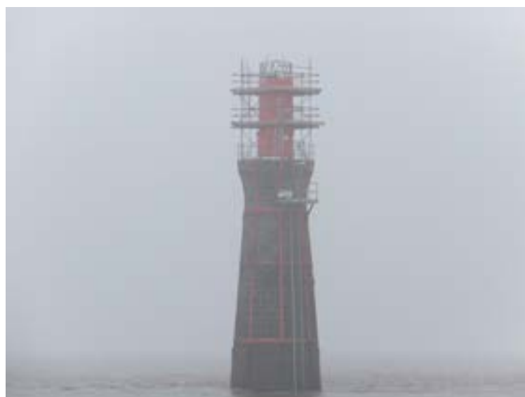
Close up of scaffolding on a misty morning.
